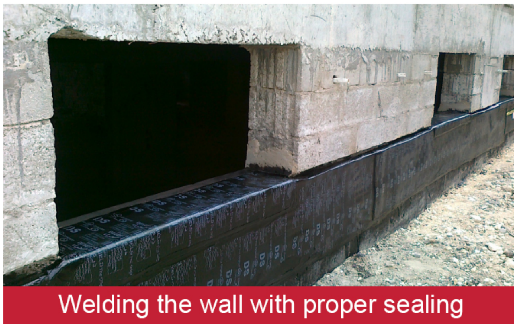
Applying bitumen on the surface
